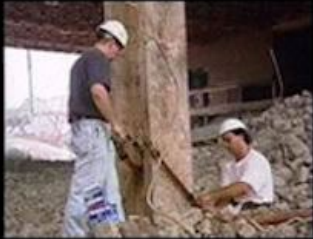
This show demolition chargers being placed on a steel column. Notice the angle of the charge. This is done to cause the building to slide or jump and collapse into it's footprint
